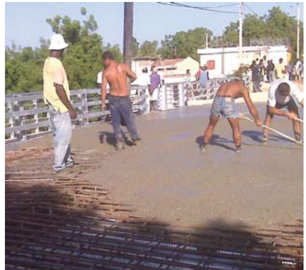
Haiti - Montrouis Bridge
