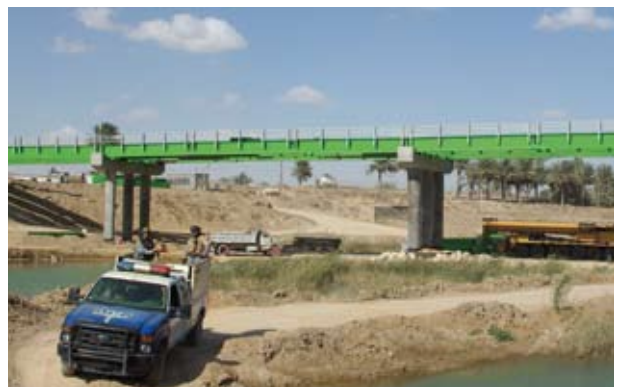
Iraq - Baghdad – Al-Nahrawan Bridge
