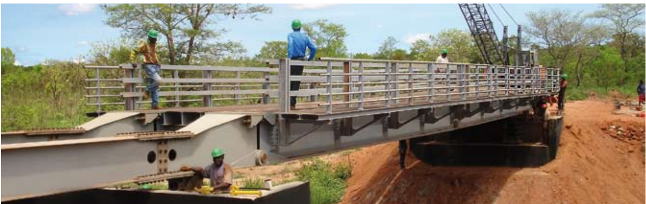
RCA - Goui Bridge
