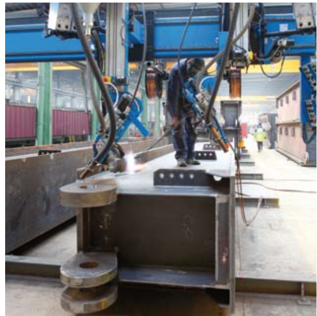
Gantry crane / finishing the box girders
