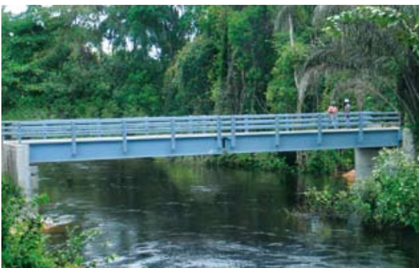
Cameroon – Bridge over the Ongue River
