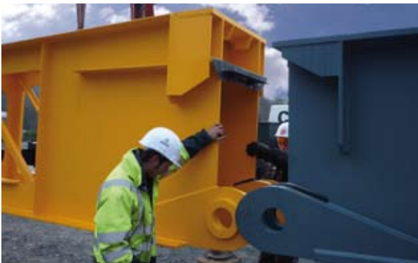
1 - Launching nose on the leading beam
