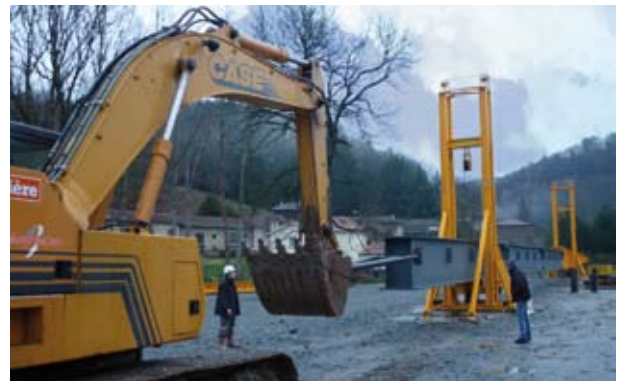
2 - Pushing with a power shovel
