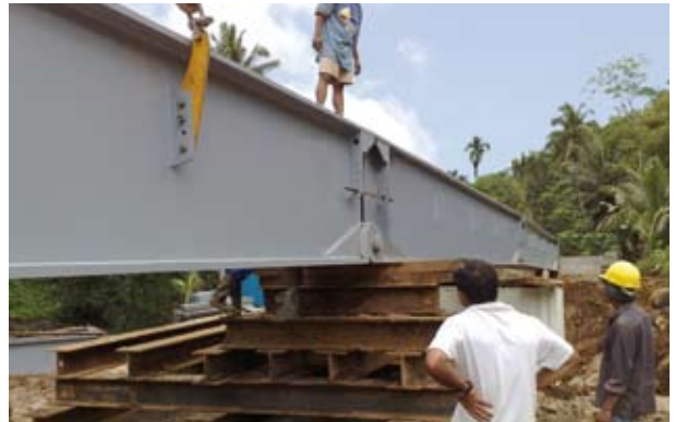
Philippines – Malibacsan Bridge
