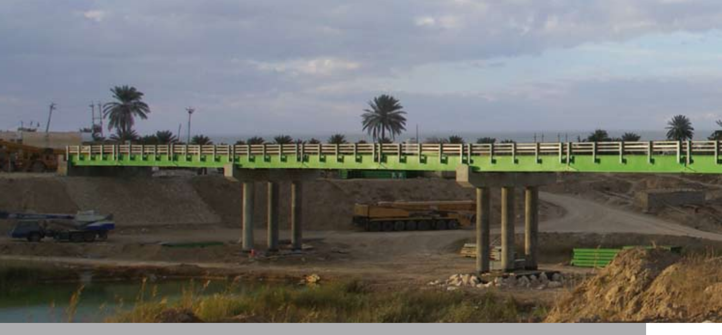
Iraq - Baghdad - Al-Nahrawan Bridge
