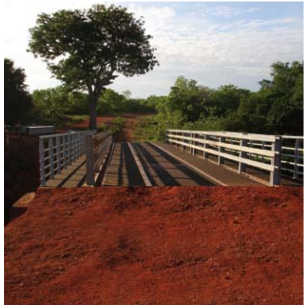
RCA - Goui Bridge
