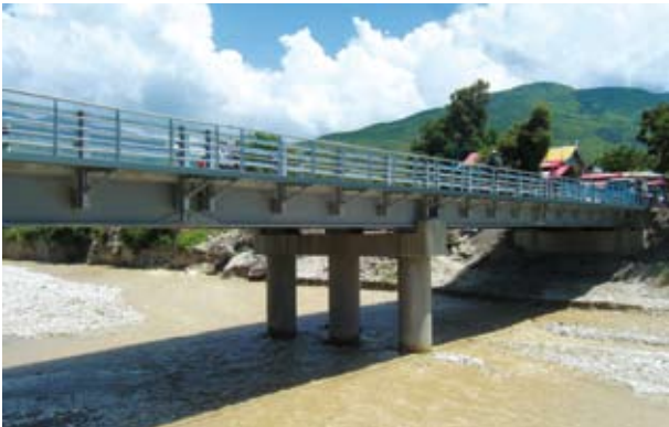
Haiti – Montrouis Bridge
