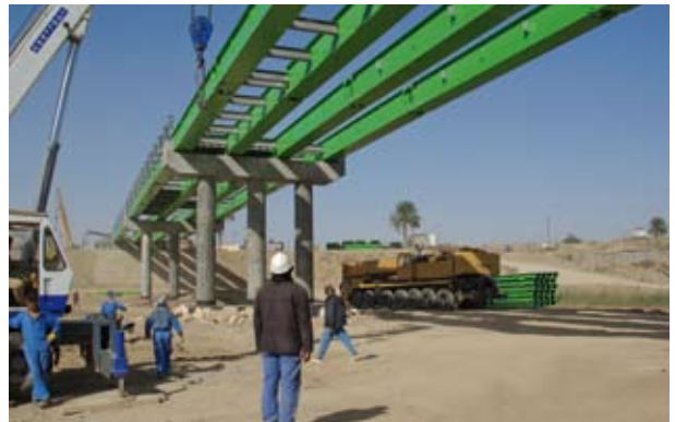
Iraq - Baghdad – Al-Nahrawan Bridge
