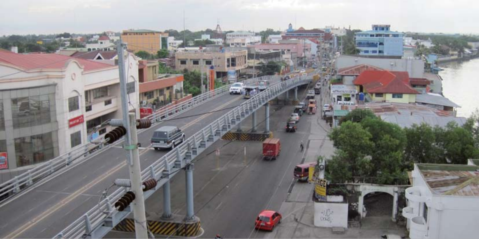
ORTHOTROPIC FLYOVER - JALANDONI FLYOVER - ILOILO - PHILIPPINES
