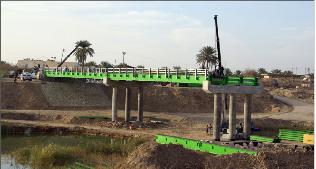
A UNIBRIDGE ® road solution built in Bagdad in 2010. The UNIBRIDGE ® Mining Solution will use the same principle for the abutments and piers.
