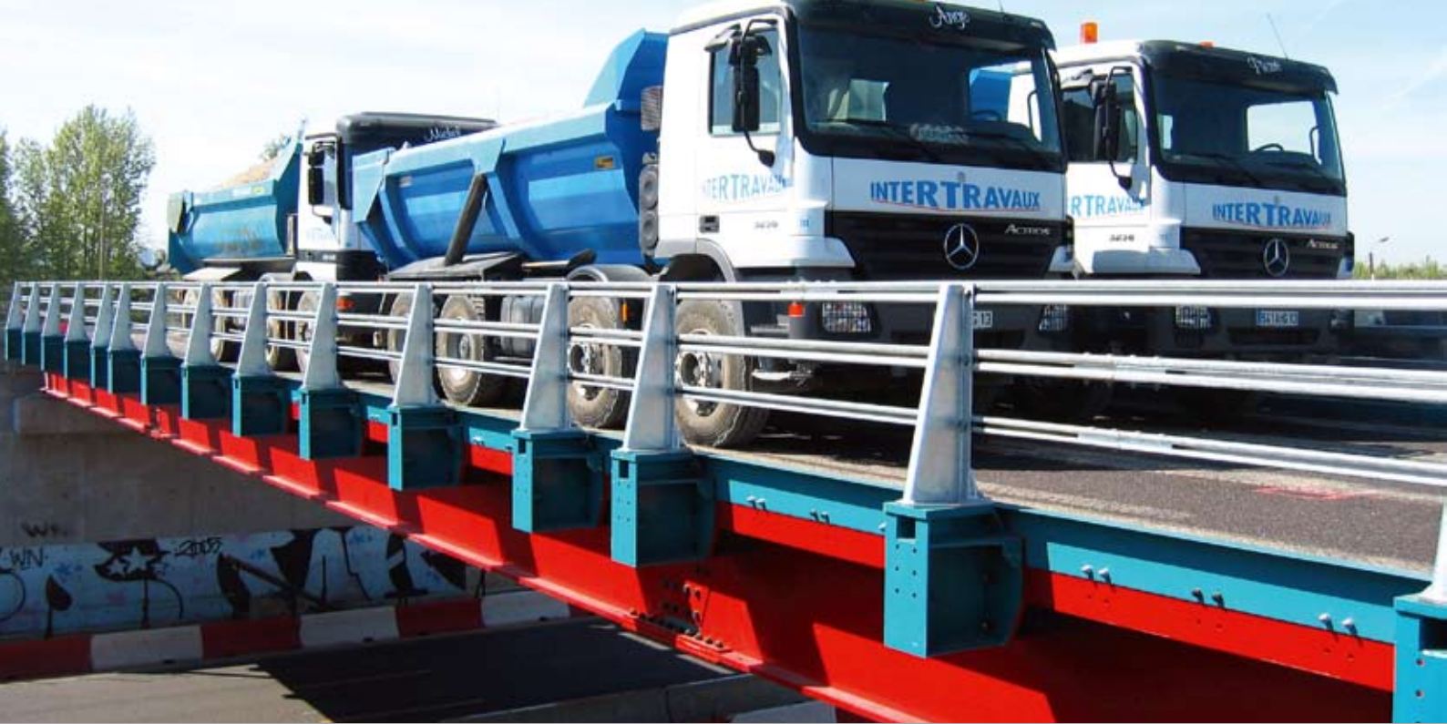
ORTHOTROPIC FLYOVER - MARSEILLE - FRANCE
